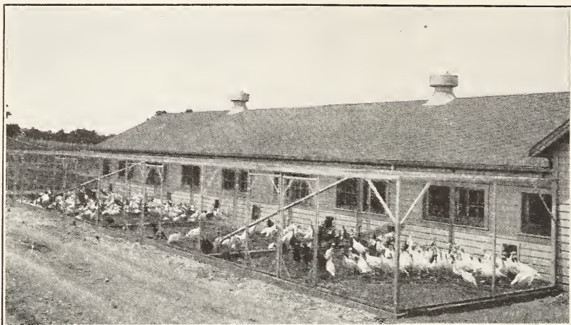
FIGURE 9.—Brooder house for raising young turkeys in partial confinement. The pens have wire floors which greatly reduce the possibility of infestation with parasites. The wire fencing extends over the top of pens to keep out sparrows and other flying birds. Electric brooders are used in each section and the building is supplied with supplementary steam heat.
